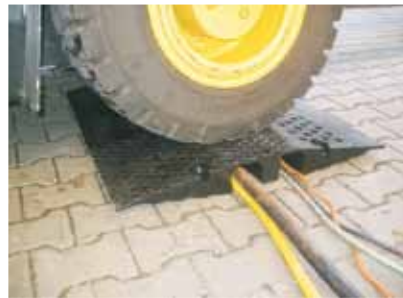
hose and cable bridge covered
